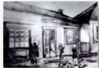
Wainwright Shop, Hindley Street
