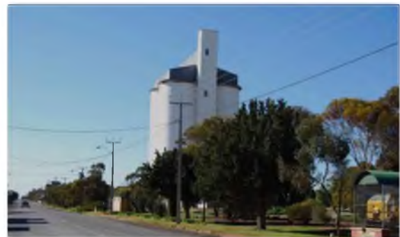
Brinkworth Silos [Source: www.panoramio.com/photo/40054352 ]
